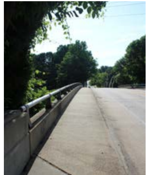
Walker Avenue bridge prior to the new railing installation.
