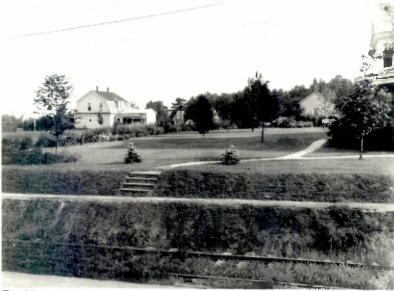
Residences Located Near a Street Car Line
